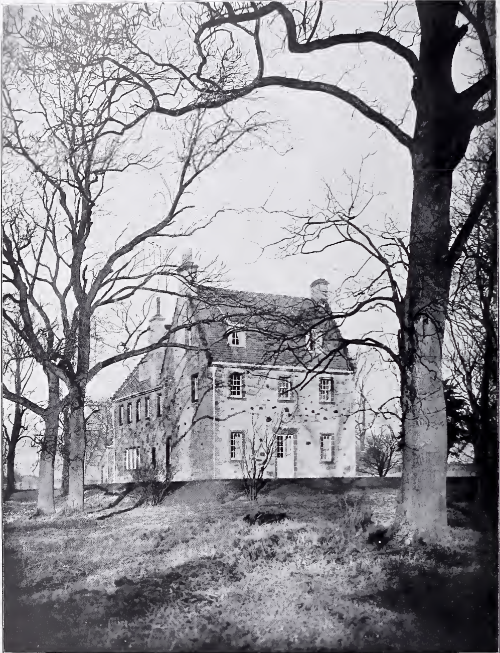
703. Boghall, Baldernock , GARDNER AND MILLAR, Architects. (For Plans, see p. 71.)
